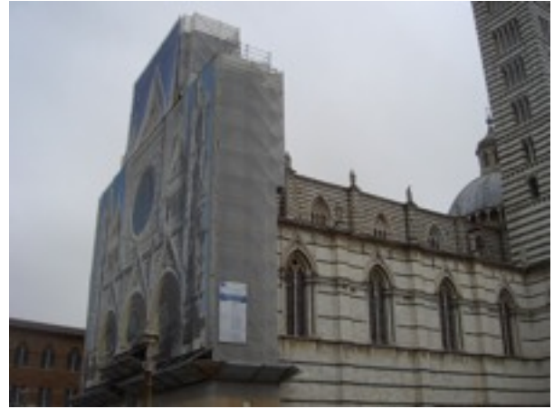
Duomo of Siena, Italy, under renovation (2006).
